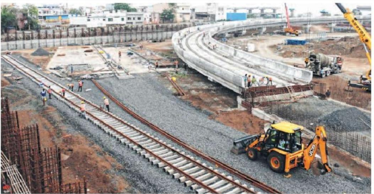
Tracks being laid down at the Metro Rail depot.
