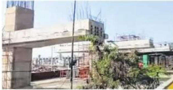
Wings of the MR10 Metro Station
