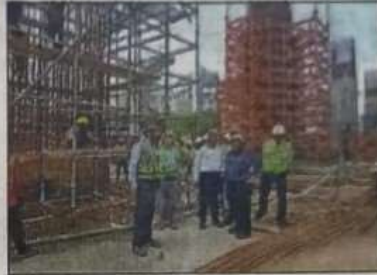
Officials led by MD, Nikunj Shrivastava inspect the Metro work underway
