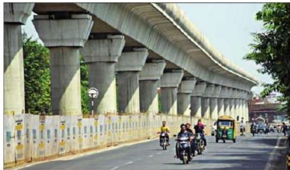
A SMOOTH RIDE: Road below elevated corridor in Indore's Vijay Nagar
