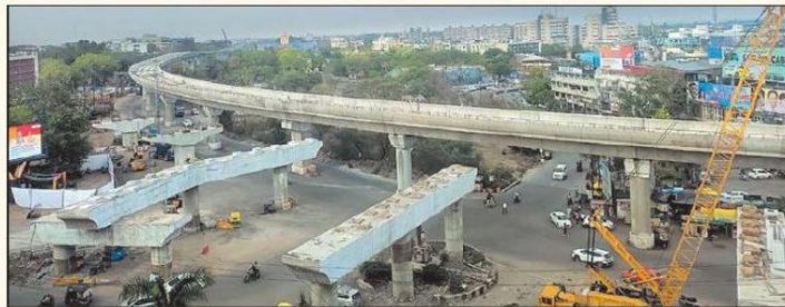
An aerial view of the ongoing work of Bhopal Metro.
