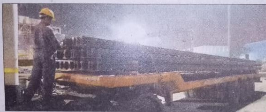
The tracks to be laid down at Subhash Nagar depot.
