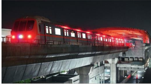
ON TRACK: Another trial run is underway for Bhopal Metro from Subhash Nagar to Rani Kamalapati railway station. Similar trial run was held in Sept year. The project is far behind schedule of the mid-2024 start announced earlier for a stretch from Depot to AIIMS Bhopal
