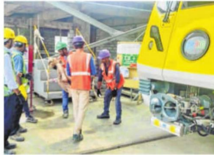
The cleanliness work done at the construction site by Metro project workers
